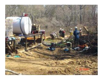
The remediation phase began the follow week; an area of oil-affected soil located between the collection station and the railroad trestle bridge was excavated. The depth of the excavation was determined by the depth and concentration of contaminants, as were indicated by the analytical results of TCEQ and Union Pacific environmental samples.
